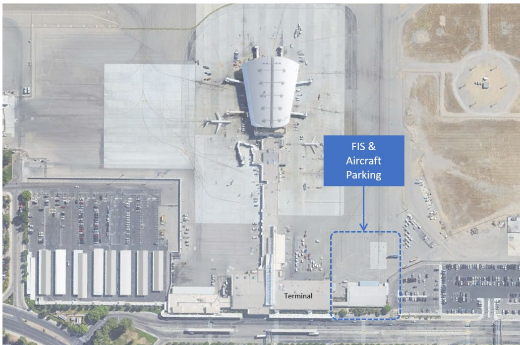
Figure 3-1. Fresno-Yosemite International Airport Existing FIS Facility Location
