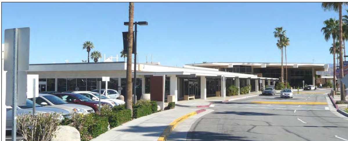
Figure 10: North end of baggage claim. View to the southeast (April 1, 2011)
