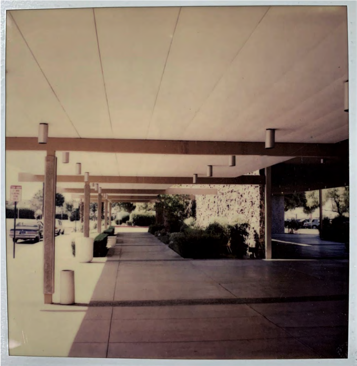
Undated poloroid photograph showing the Granulux columns supporting the canopy along the southwest elevation.
