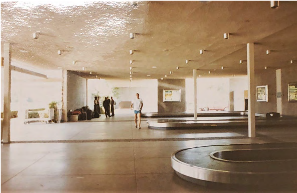
Baggage claim area (open air) prior to being enclosed. Source: Palm Springs Art Museum Architecture and Design Center.
