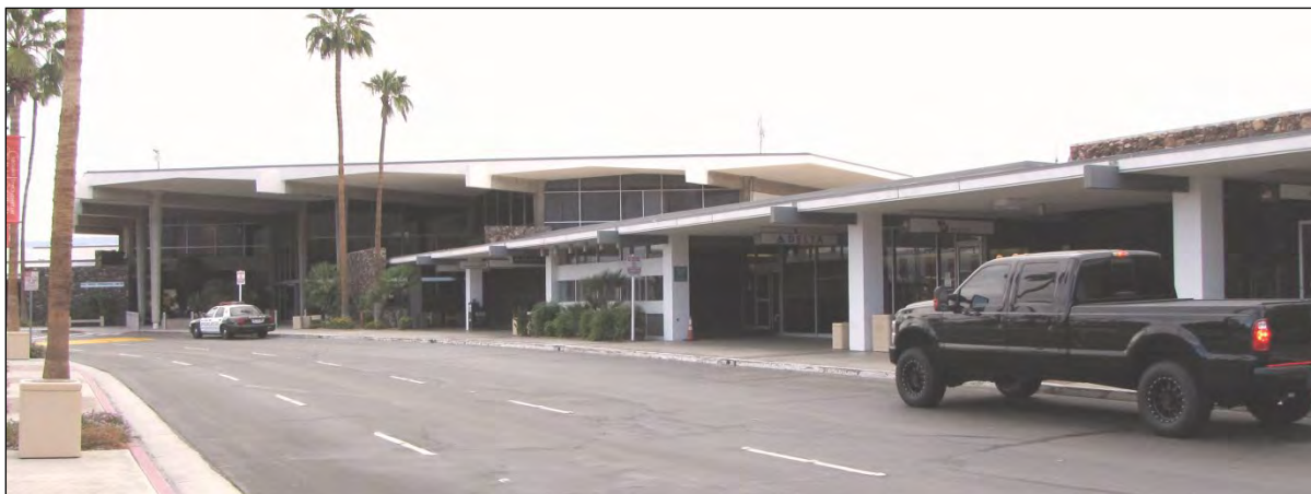
Figure 12: Main entrance and ticketing area. View to the northeast (November 7, 2012)
