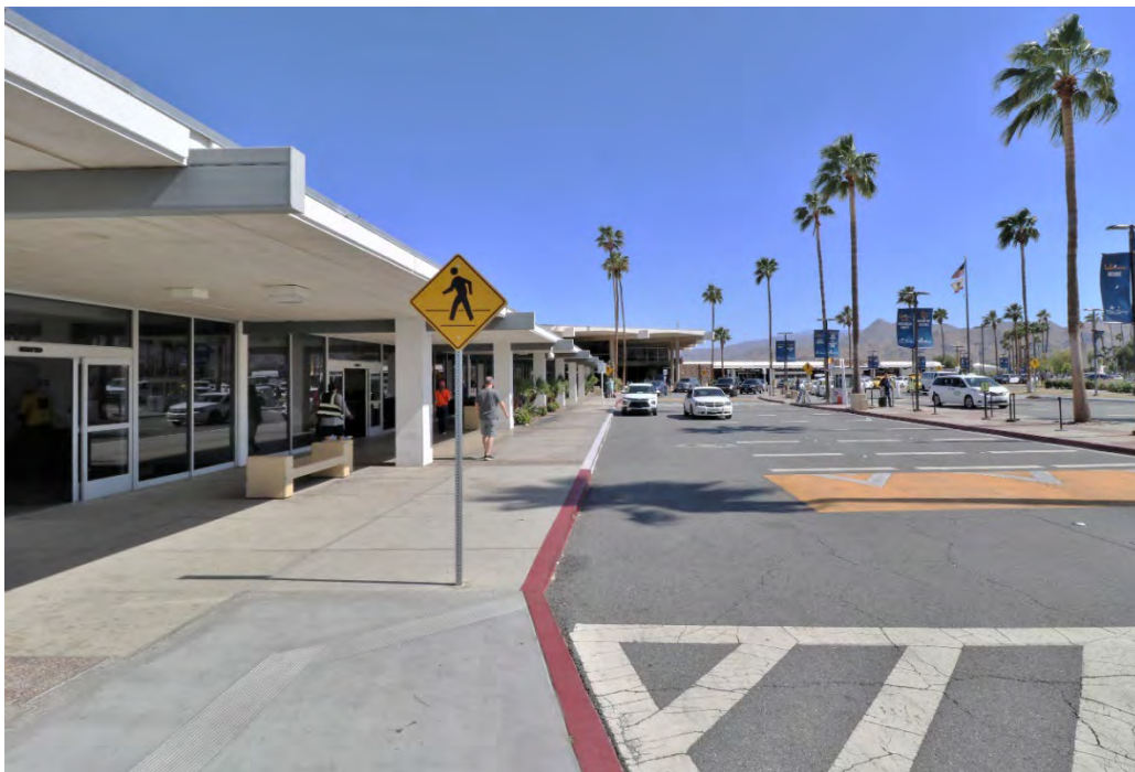
Canopy and southwest elevation of baggage claim area, view southeast (4/17/23).
