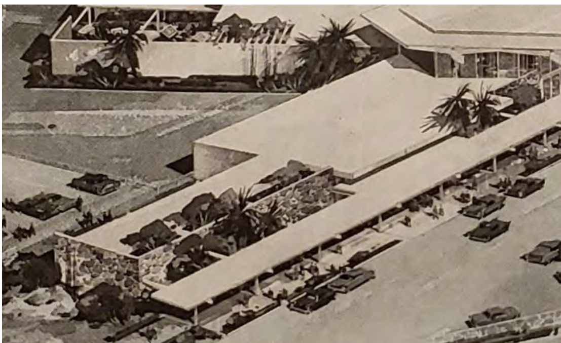
Detail showing the open air baggage claim area in the northwest wing of the terminal.
