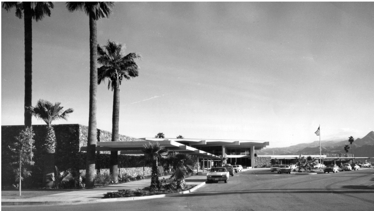
Northwest end of terminal building prior to any additions. Source: Palm Springs Art Museum Architecture and Design Center.
