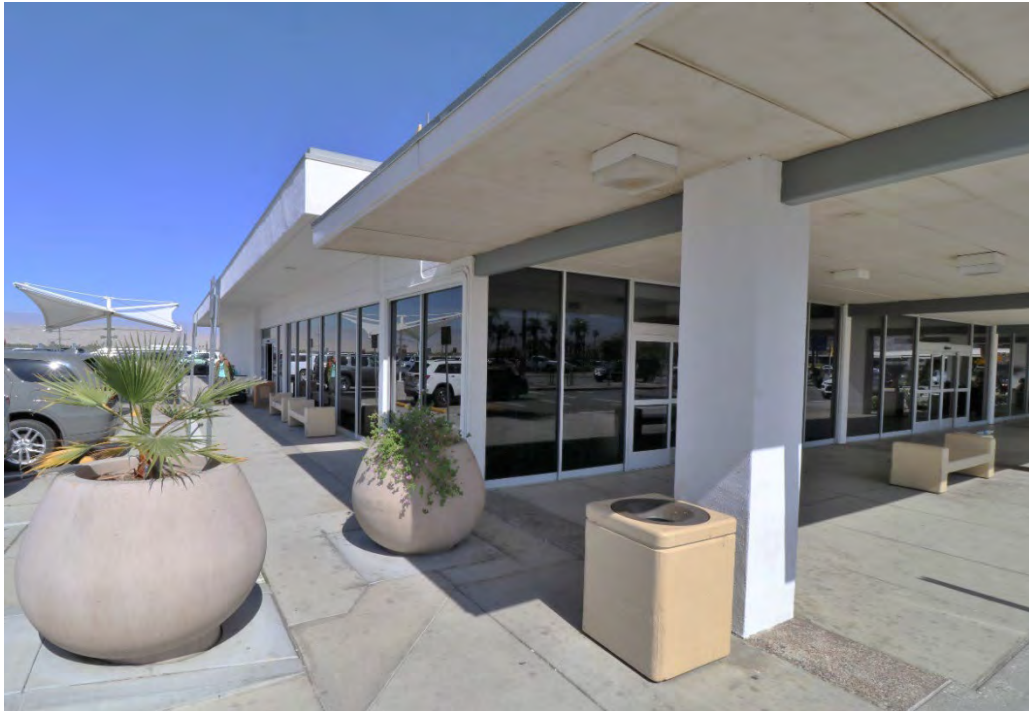
Northwest corner of the baggage claim area, view east (4/17/23).
